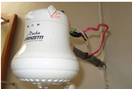
Figure 20.44 On-demand electric hot water heater. Heat is supplied to water only when needed. (credit: aviddavid, Flickr)
