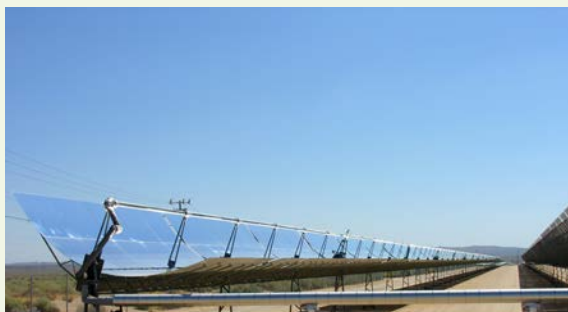
Figure 25.43 Parabolic trough collectors are used to generate electricity in southern California. (credit: kjkolb, Wikimedia Commons)
