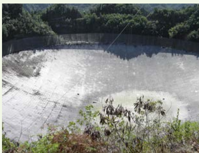
Figure 27.28 A 305-m-diameter natural bowl at Arecibo in Puerto Rico is lined with reflective material, making it into a radio telescope. It is the largest curved focusing dish in the world. Although D for Arecibo is much larger than for the Hubble Telescope, it detects much longer wavelength radiation and its diffraction limit is significantly poorer than Hubble's. Arecibo is still very useful, because important information is carried by radio waves that is not carried by visible light. (credit: Tatyana Temirbulatova, Flickr)
