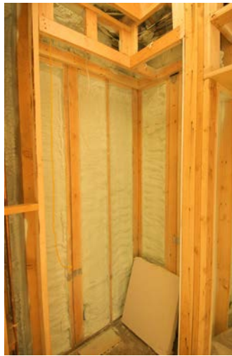
Figure 14.13 Insulation is used to limit the conduction of heat from the inside to the outside (in winters) and from the outside to the inside (in summers). (credit: Giles Douglas)
