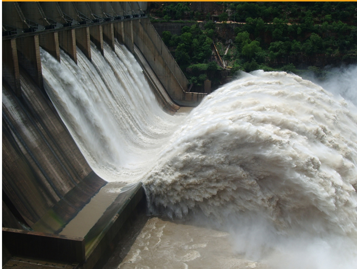
Figure 20.1 Electric energy in massive quantities is transmitted from this hydroelectric facility, the Srisaïlam power station located along the Krishna River in India ( http://en.wikipedia.org/wiki/Srisaïlam_Dam ), by the movement of charge—that is, by electric current. (credit: Chintoher, Wikimedia Commons)
